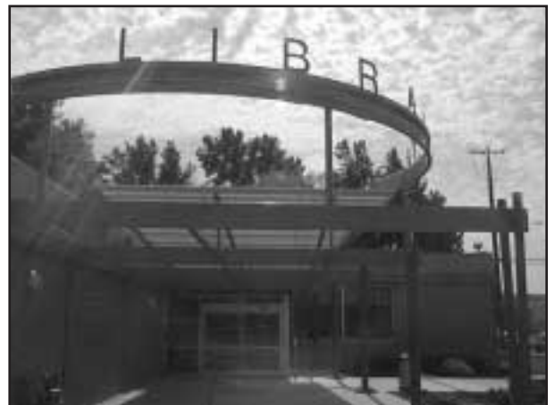
Keewaydin Park Branch entrance walkway, door area, and sign.
